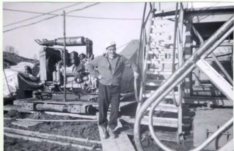
A close-up view of the rig.
