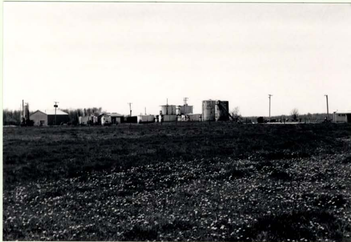
This is the Cowal Oil Battery where the oil from all the wells is collected, then taken to Sarnia by truck to be refined. The Battery is located on the farm of Robert Murray. (June 1984)
